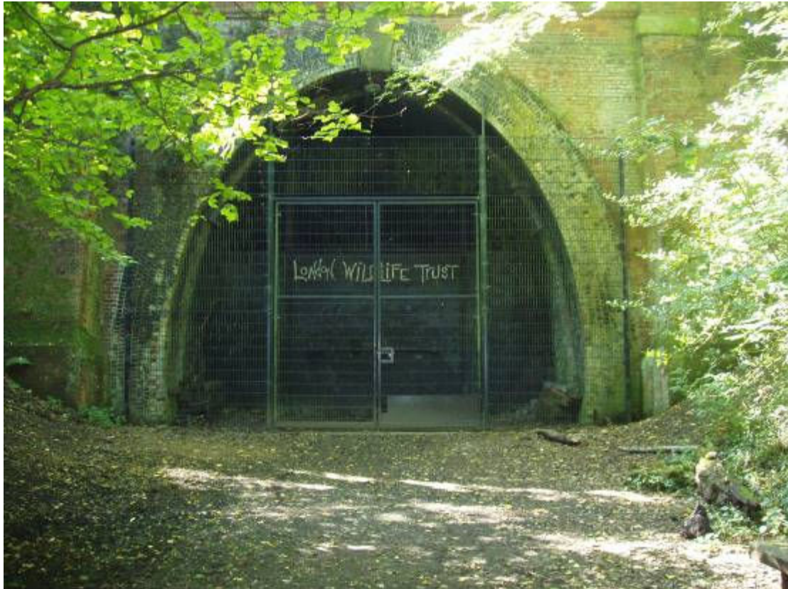
Entrance to the railway tunnel in Sydenham Hill Wood LNR (Now a bat registered roost).
